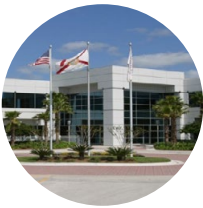
Building demolition and renovation
