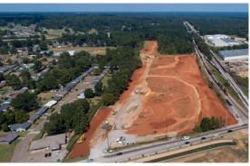
Over 110,00 tons of creosote contaminated soil excavated 91 tons of wooden railroad ties removed
