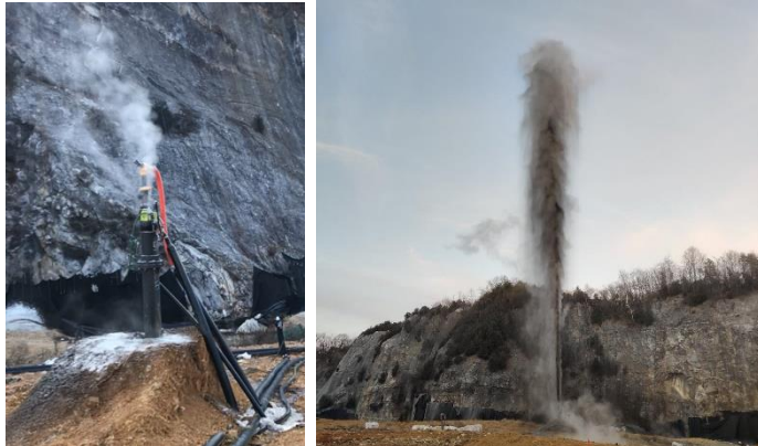
Left: Hot gas escaping from a landfill gas collection well. Right: A geyser of hot liquid from deep within the landfill. Source: City of Bristol, VA.
