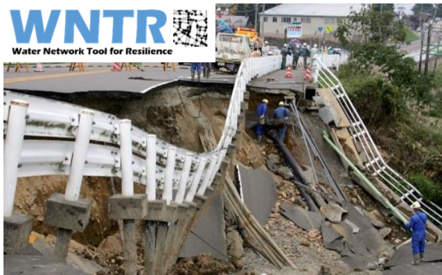
Figure 1: Damage following earthquake, including broken pipes.
