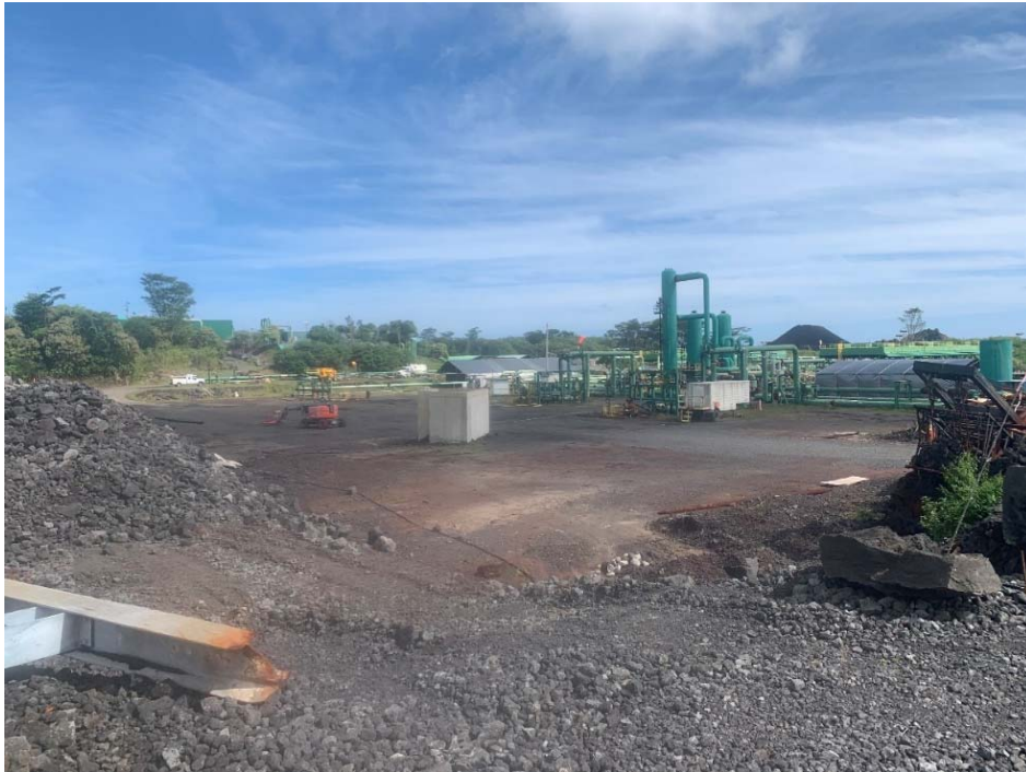
Example of Well Pad Conditions
