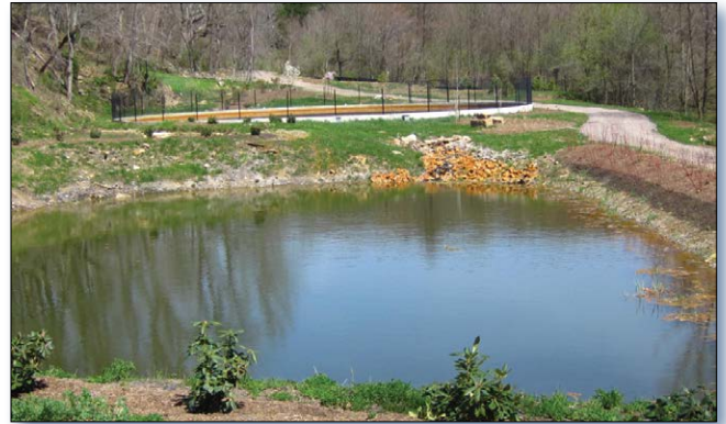
Figure 2. The Owens South AMD mitigation site includes an oxidizing pond (foreground) and successive alkalinity-producing system cells (background).
