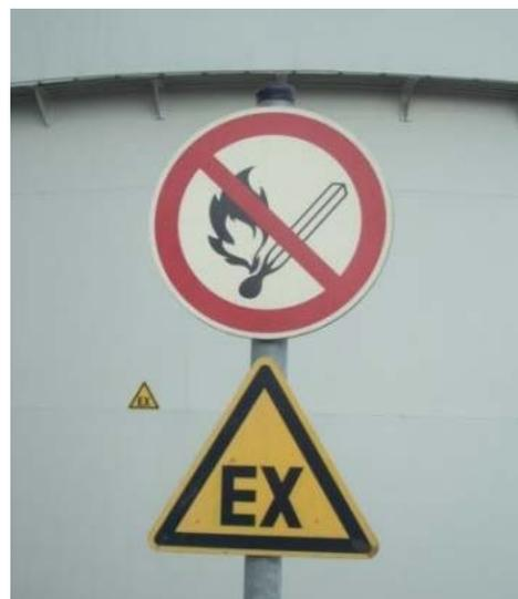
**Figure 10-2. Explosion potential sign.** <sup>24</sup>
