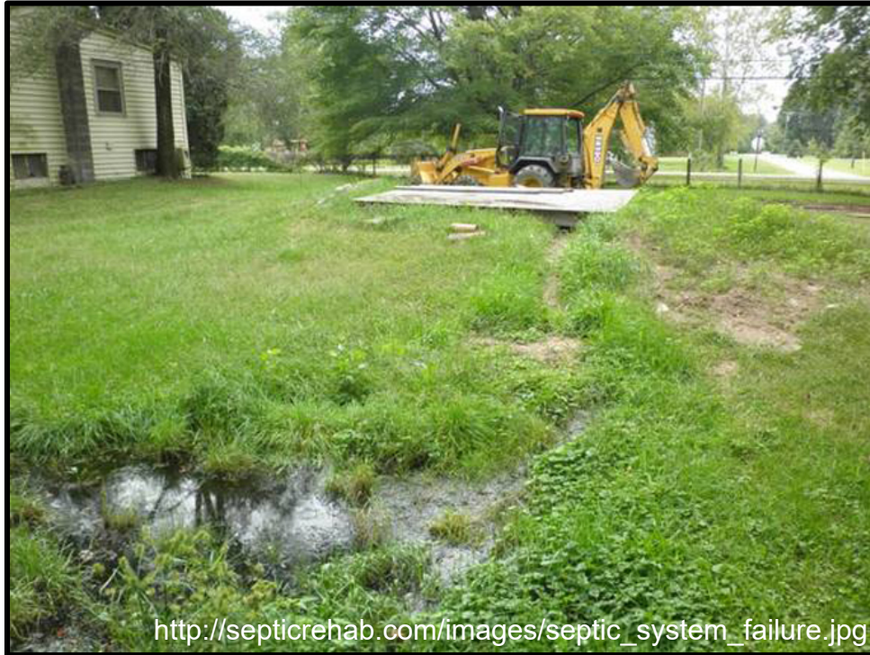
Failing septic system
