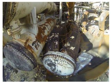
Figure 3 Reboiler, post-accident
