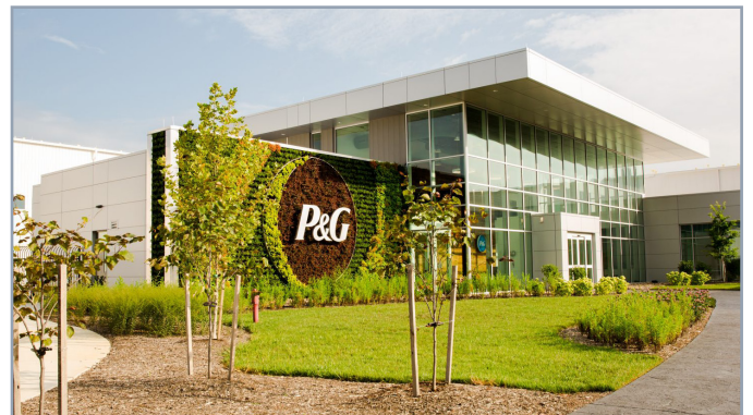
Living wall at the entrance of the Proctor and Gamble Tabler Station Plant.
