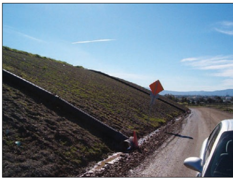
Figure 9. Slope drains to protect a hillside from erosion.
