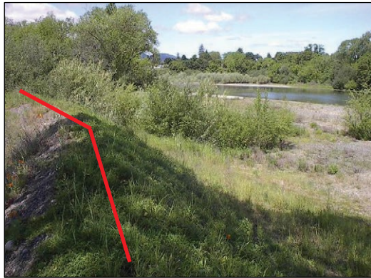
Figure 10. Vegetated berm used to prevent facility inundation when the river is at flood stage.
