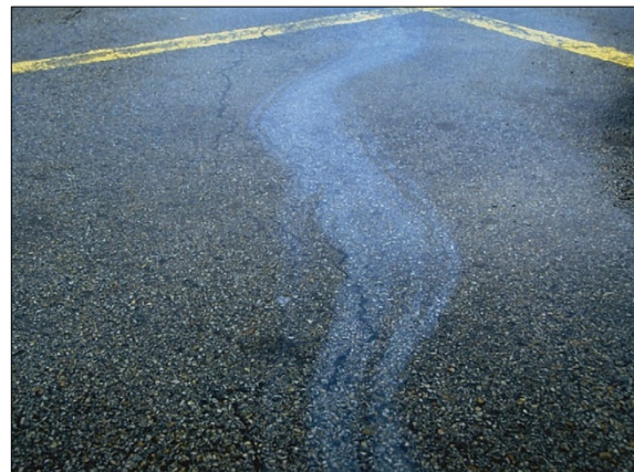
Figure 14. Example of a sheen indicating the presence of oil or other hydrocarbons.
