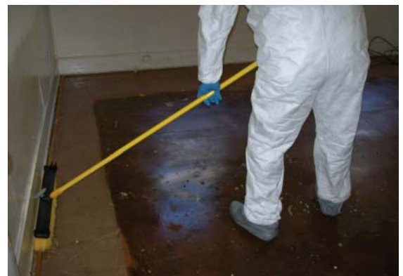
Scrubbing the walls and baseboards with the Sterilex® solution
