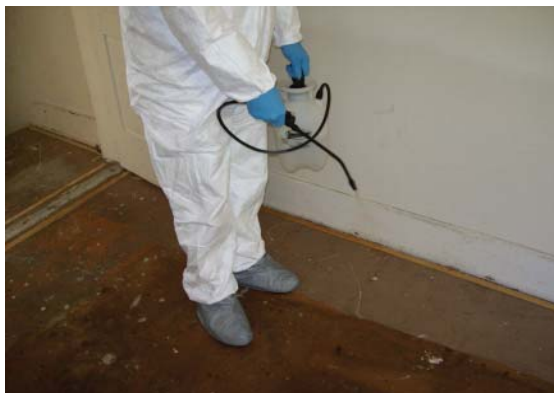
Pre-soaking the walls and baseboards
