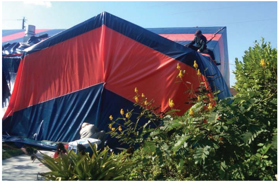
During an exercise in Florida, a structure is tented prior to fumigation with methyl bromide
