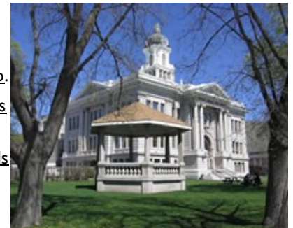
Missoula County received a $279,000 multipurpose grant to conduct asbestos assessment and cleanup at Missoula County Courthouse. Photo Courtesy of Missoula County.
