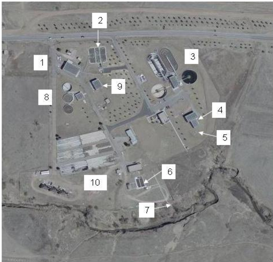
Figure 1 Aerial View of Fort Carson Sanitary Wastewater Treatment Facility
