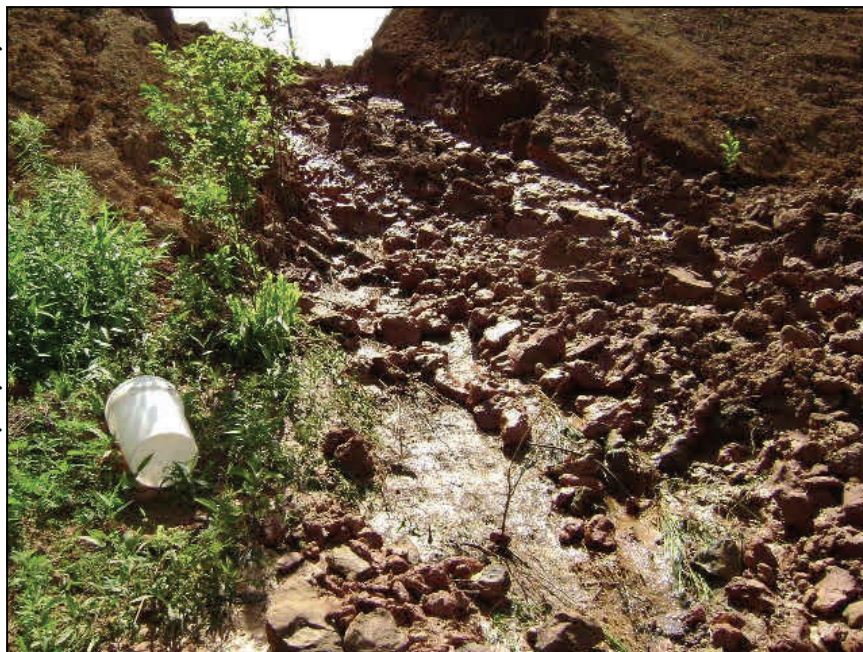
Photograph taken from the backside of the reservoir. It shows the breach and the slope of the terrain.
