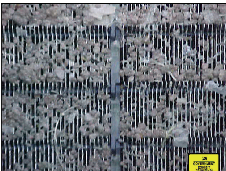
The bar screen at the City of Raeford's POTW contaminated with turkey parts / turkey solids.
