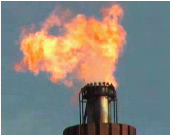
Well Operating Flare – High Combustion Efficiency
