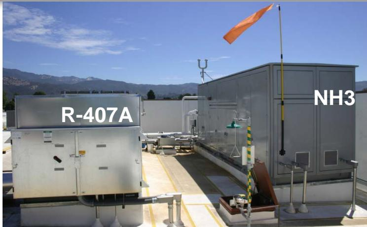
**The Carpinteria refrigeration system is a Cascade design with CO<sub>2</sub> as the in-store refrigerant:**
