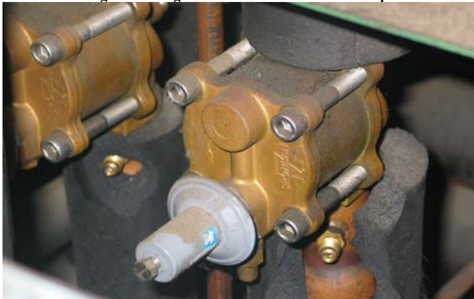
Figure 3: Image of a Schrader valve with no caps
