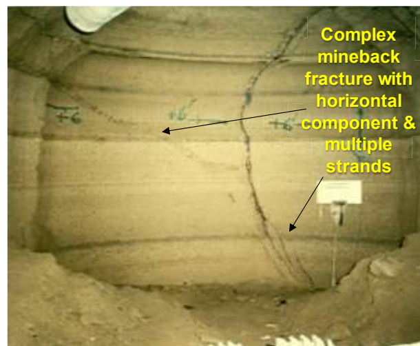
Figure 12. Mineback photograph of complex fracture
