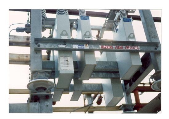
Figure 2. Looking up at PCB Marked Capacitor on the left
