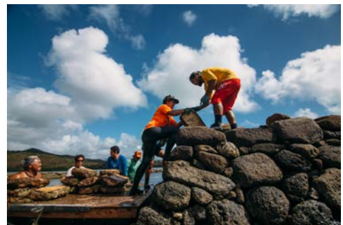
Community members come together to restore the walls of a traditional Hawaiian fishpond. (Photo courtesy of KUA)
