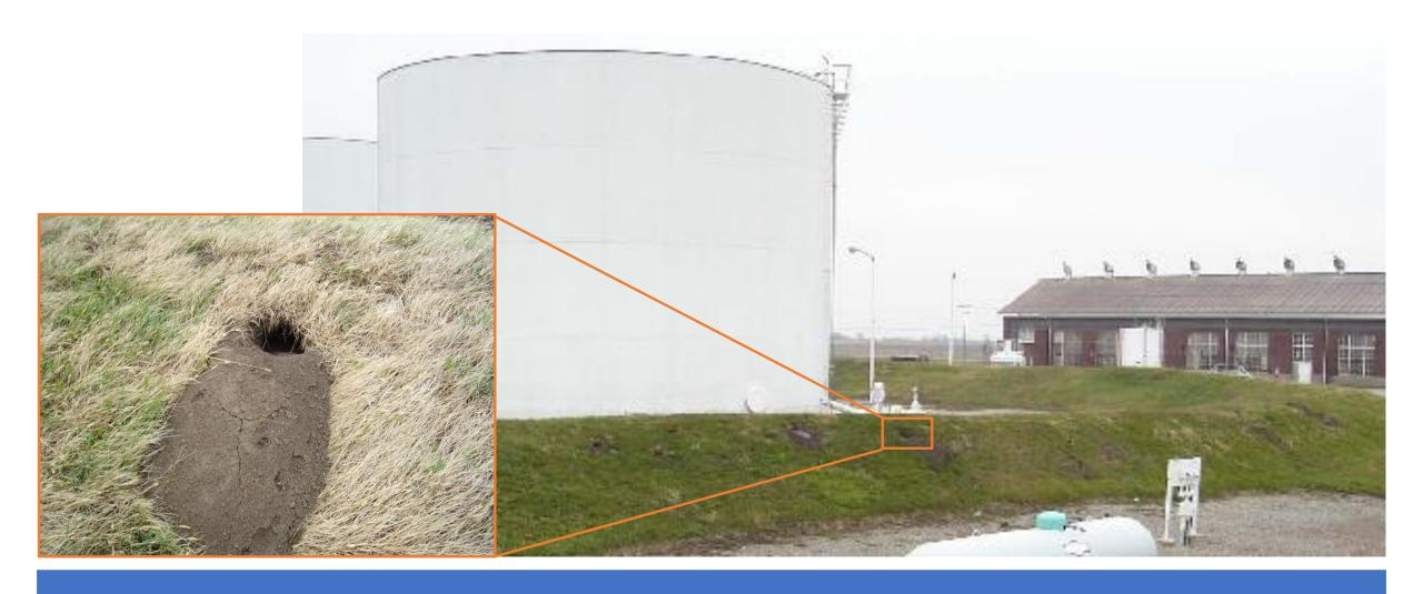
Erosion and animal burrowing through the containment wall renders the berm ineffective at containing oil.
