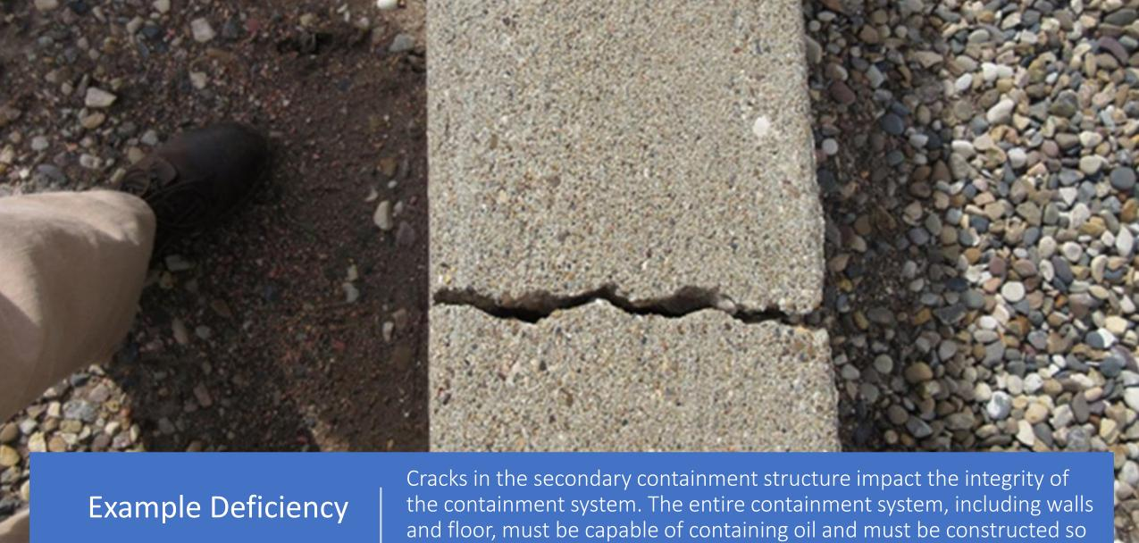
that any discharge from a primary containment system, such as a tank, will not escape the containment system before cleanup occurs.
