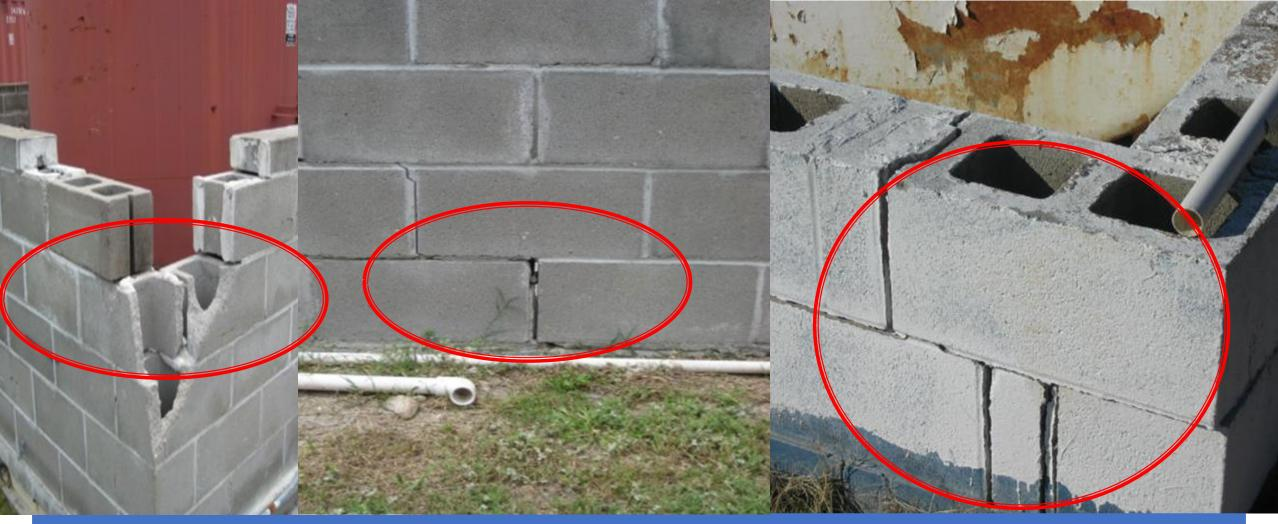
Concrete block failure and damage impacting secondary containment integrity. The entire containment system, including walls and floor, must be capable of containing oil and must be constructed so that any discharge from a primary containment system, such as a tank, will not escape the containment system before cleanup occurs. Additionally, concrete block dikes need to be sufficiently impervious to contain discharged oil.
