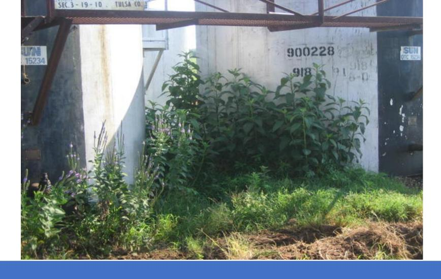
It would be very difficult for the owner operator of this production facility to complete visual inspections given excessive vegetation limiting visibility to the tanks.
