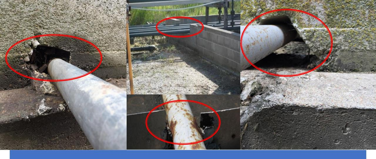
Dike wall penetrations must be engineered such that oil can't escape. Situations like those depicted above may lead to a significant reduction in the secondary containment dike capacity relative to the height of the pipe penetration where oil may escape.
