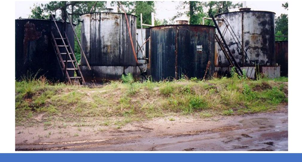
Production transfer area appears to lack adequate general secondary containment.
