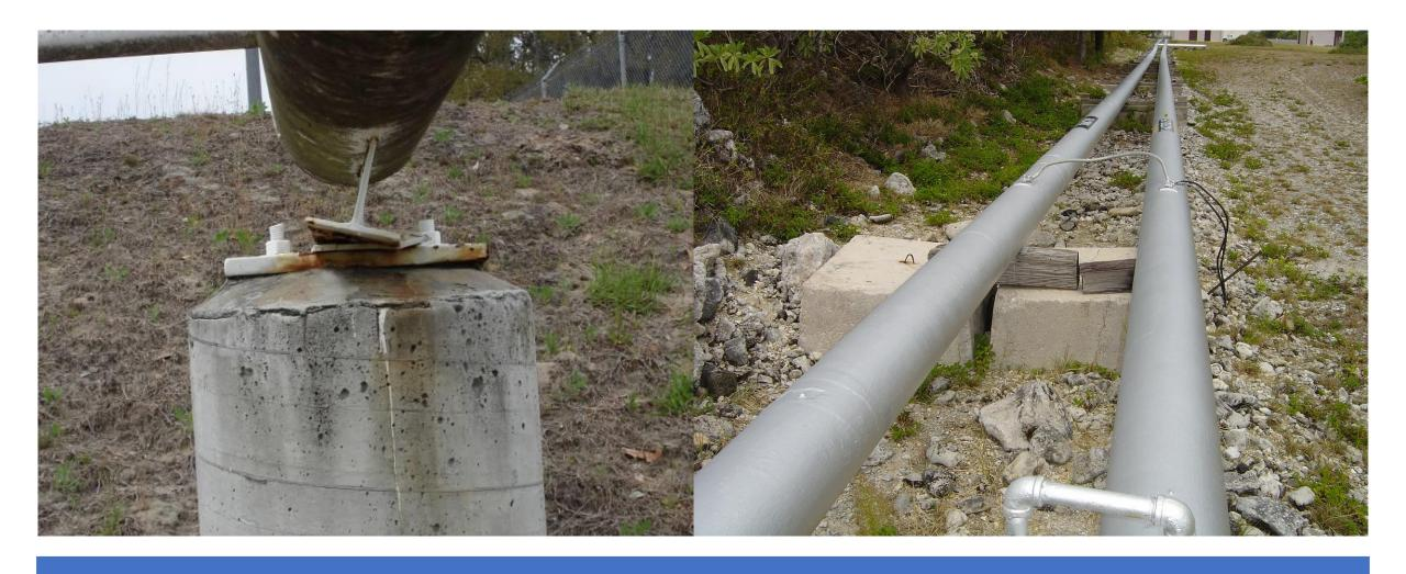
Pipe supports are inadequate and not designed to minimize abrasion and corrosion.
