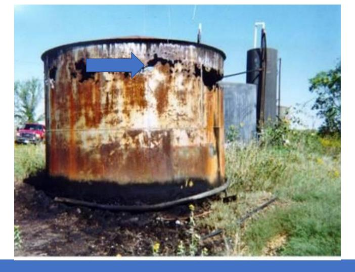
There appears to be no regular schedule to visually inspect each container of oil for deterioration and maintenance needs, including the foundation and support of each container that is on or above the surface of the ground.
