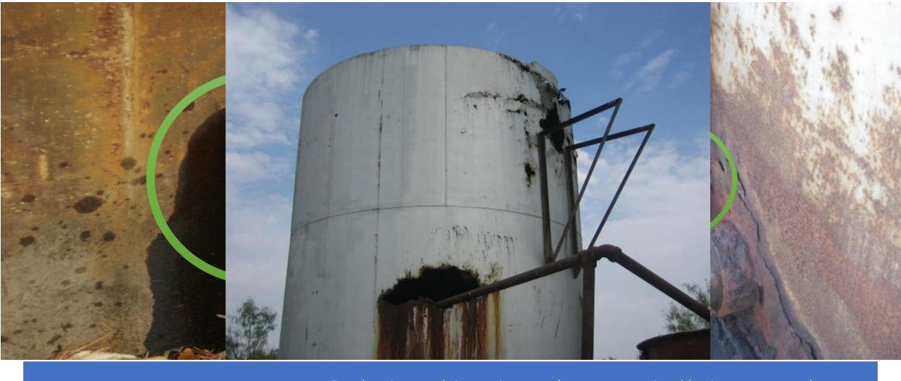
Production tank integrity may be compromised by improper tank repairs or alternations which may not be in accordance with industry standards, recommended practices, design specifications or good engineering practices.
