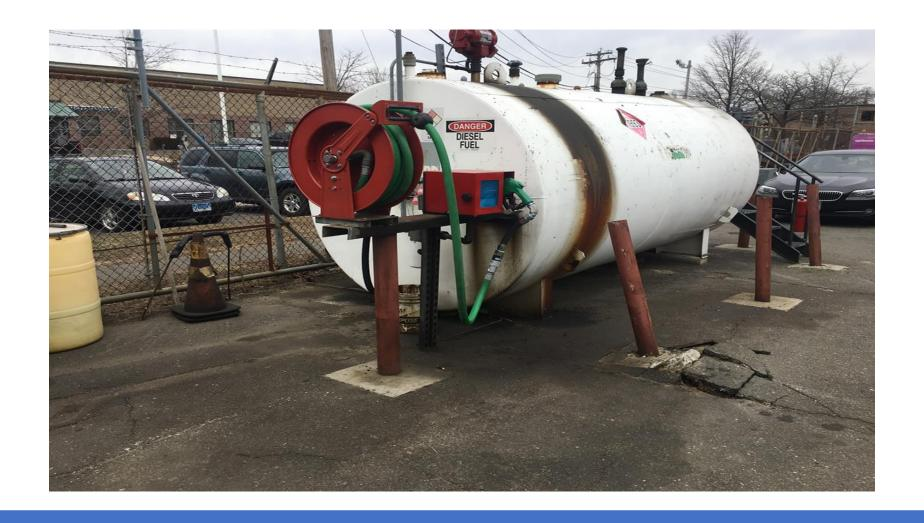
Often, EPA finds general containment for transfers and vents associated with double walled tanks not addressed in the Plan and/or not implemented in the field.
