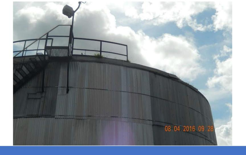
Vegetation at the top of the tank may indicate water collection inside tank's insulating jacket. The facility's routine tank integrity visual inspection program appears to be flawed.
