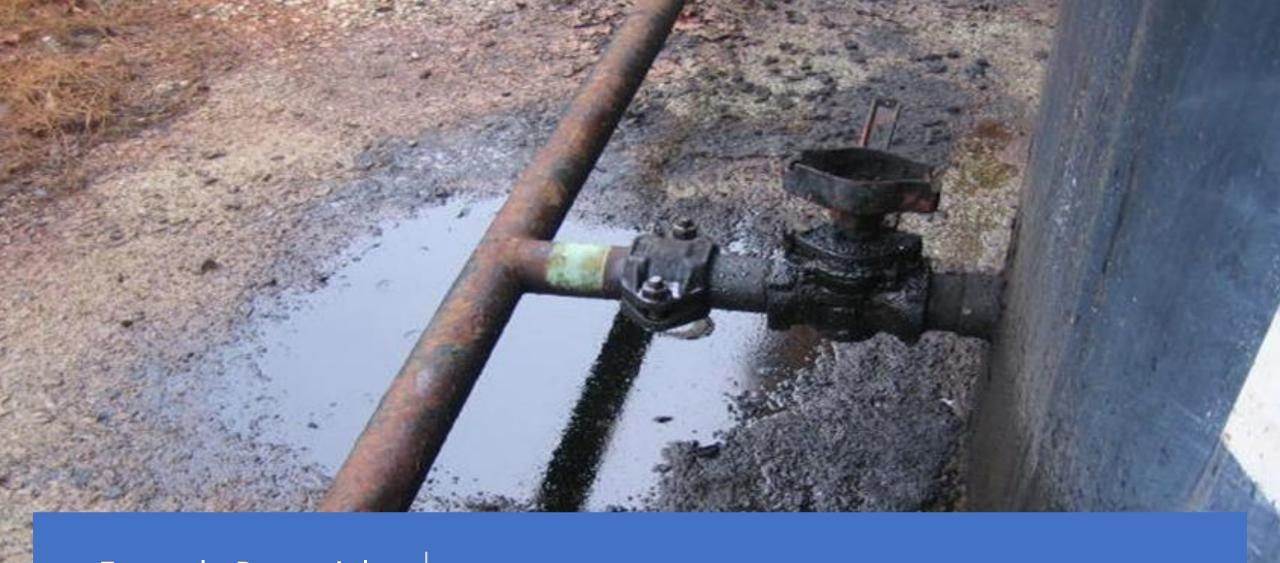
Leaking piping and valves. Inspection program is questionable.
