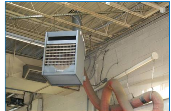
Infrared Heater - Lorton, VA
