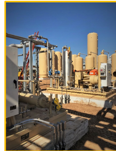
RNG Plant – Phoenix, AZ
