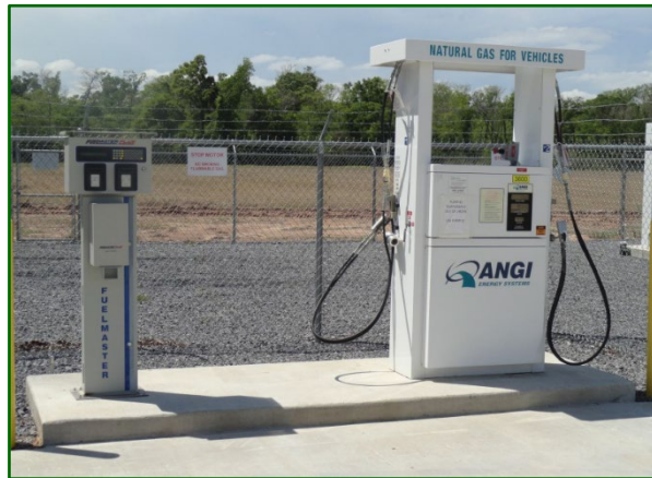
CNG Fueling Station St. Landry Parish, LA
