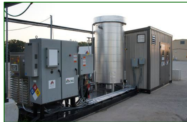
BioCNG System Dane County, WI
