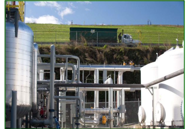
RNG Pipeline Project Rochester, NH
