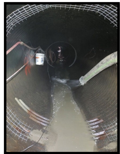
Down-flow discharge area
