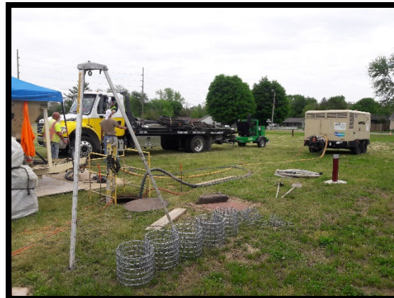
View of compressor for shotcrete application
