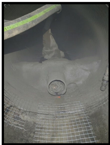
Temporary weir and pump intake
