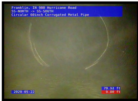
Overall visual separation of joint
