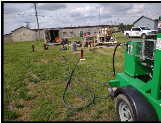
View of dewatering pump and shotcrete mixing equipment
