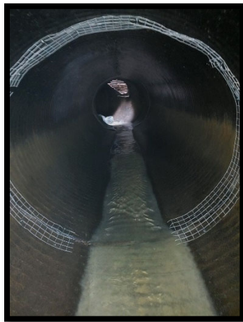
View of wire mesh at joint
