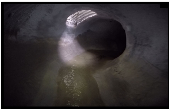
View of repaired main turn at SS-North
