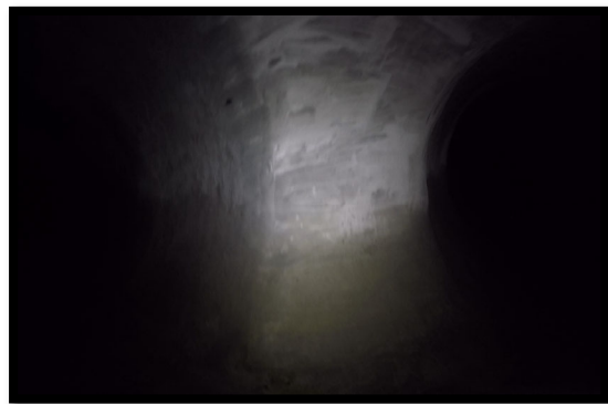
View of repaired main turn at SS-South (Northeast corner)
