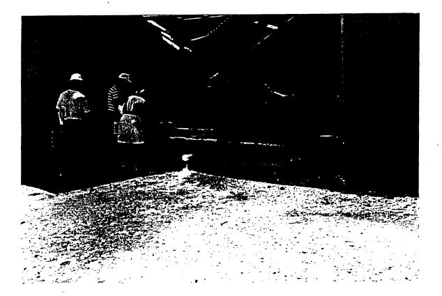
Date: <u>08/23/93</u> Picture Taken by: <u>K. Matherne</u> Direction Facing: <u>Northwest</u> Picture Description: <u>Above-grade concrete tank in the former water treatment area (SWMU No. 6);</u> note the white crystalline powder in the pipe protruding from the side of the wall (center of photograph).
