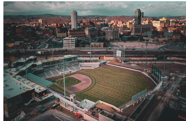
Aerial View of Polar Park. (photo credit City of Worcester)
