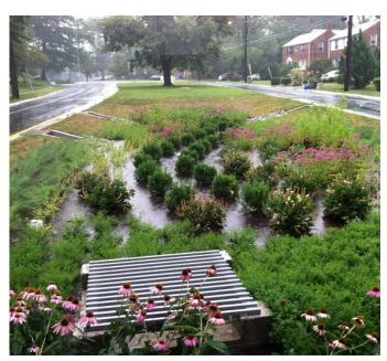
A bioretention practice in a suburban road median, capturing stormwater during a rain event. Photo Credit: Image reproduced with permission from Montgomery County, MD Department of Environmental Protection
