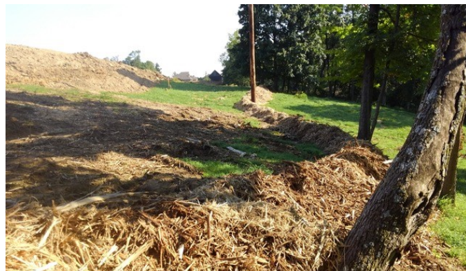
A brush barrier at the perimeter of a construction site. Credit: Hamilton County Soil & Water Conservation District
