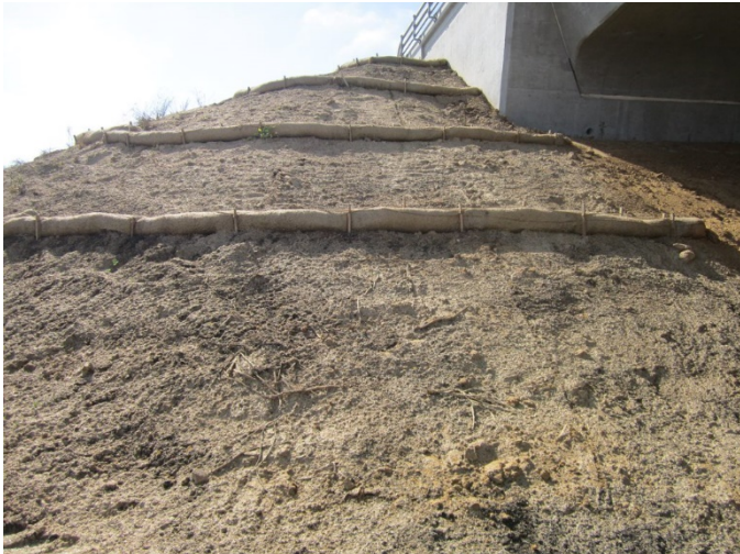
Fiber rolls can control erosion when installed perpendicular to the slope and spaced appropriately.
