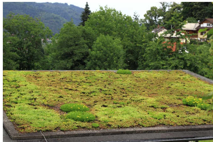
Green roofs provide an opportunity to utilize traditionally unused spaces for stormwater management
