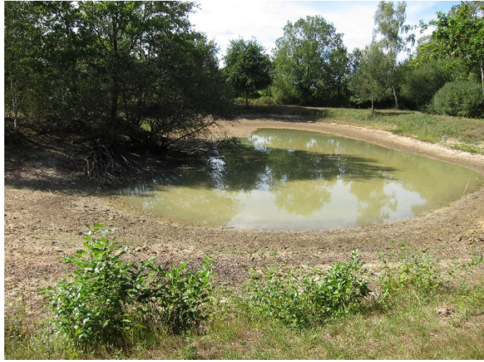
Infiltration pond in a natural area. The infiltration portion consists of sand with a high infiltration rate.
