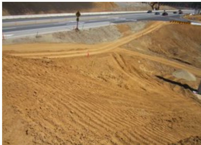
Land grading involves reshaping the ground surface to planned elevations.
