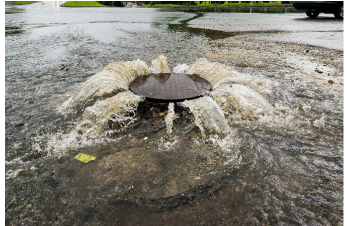
Sanitary Sewer Overflows can contribute significant pollutants to stormwater when not properly addressed.
