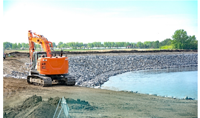
A riprap-lined bank surrounding a newly constructed detention pond.
