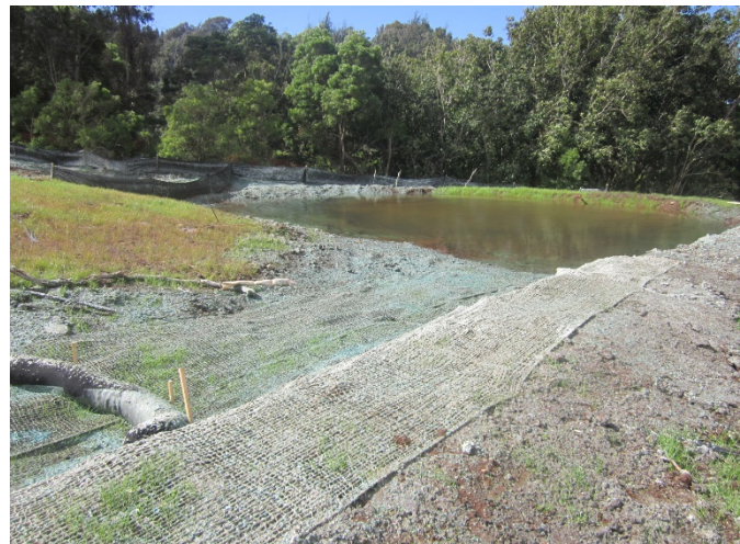
A sediment basin with earthen embankments stabilized with erosion matting and hydroseed.
