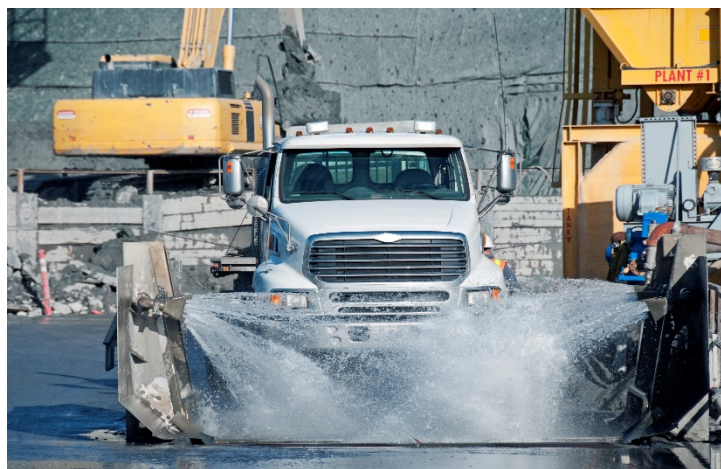
A truck having its tires washed before leaving a construction site.
