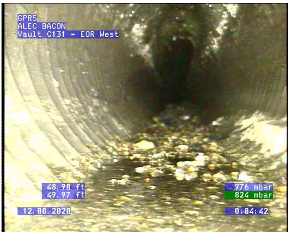
Vault C131 - EOR West_0006.bmp, , 48.92ft Deposits Settled Gravel, 5% of cross sectional area from 5 o'clock, Start
