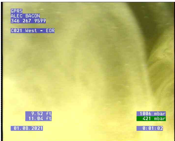
C021 West - EOR_0001.bmp, , 9.51ft Camera Underwater
