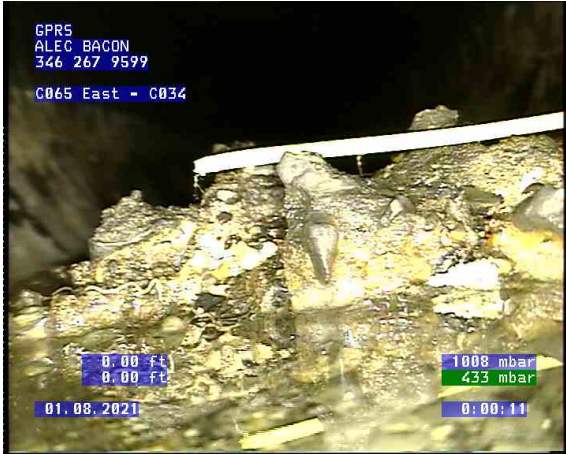
C065 East - C034_0000.bmp, , 0.00ft Water Level
