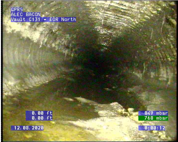
Vault C131 - EOR North_0001.bmp, , 0.00ft Water Level
