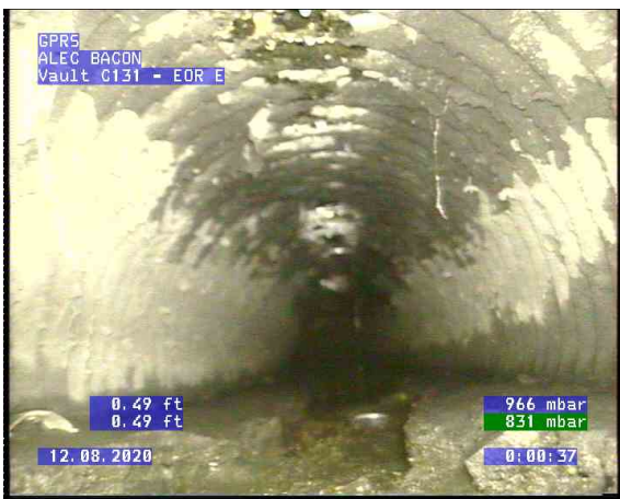
Vault C131 - EOR E_0002.bmp, , 0.49ft Survey Abandoned / could not make it past obstruction
