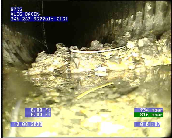
CB C065 - Vault C131_0002.bmp, , 0.00ft Deposits Settled Compacted, 10% of cross sectional area from 5 o'clock to 7 o'clock, Start
