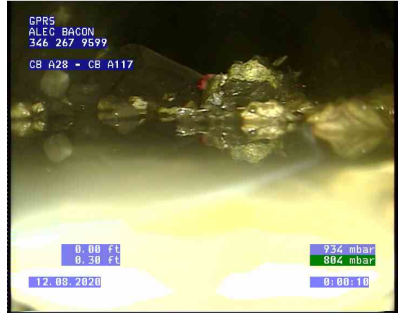
CB A28 - CB A117_0001.bmp, , 0.00ft Water Level
