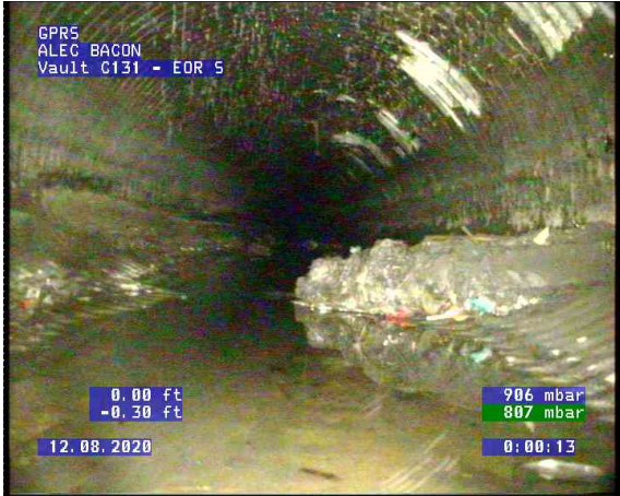
Vault C131 - EOR S_0001.bmp, , 0.00ft Water Level
