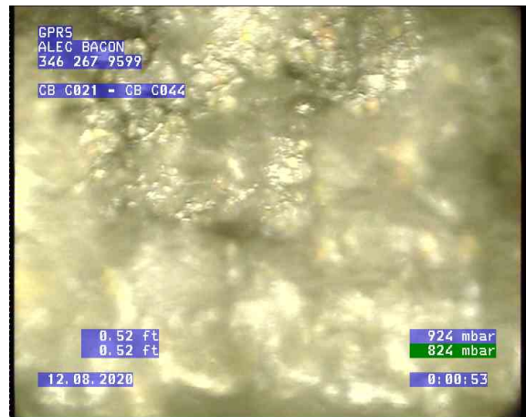
CB C021 - CB C044_0003.bmp, , 0.52ft Dye Test Visible / could not make it past deposit
