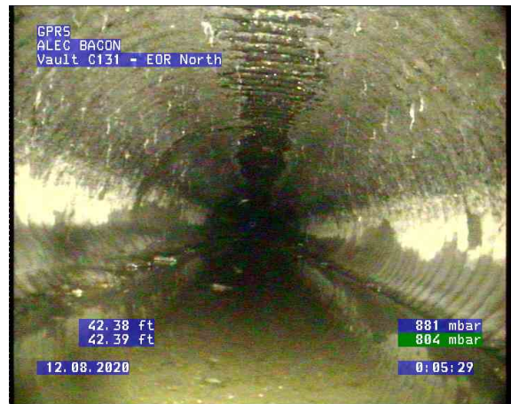
Vault C131 - EOR North_0003.bmp, , 42.39ft Survey Abandoned / could not make it, slick surface
