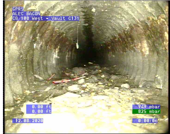
CB C108 West - Vault C131_0001.bmp, , 0.00ft Catch Basin
