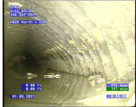
A028 North - EOR_0001.bmp, , 0.00ft Deformed, 10% changed, Start
