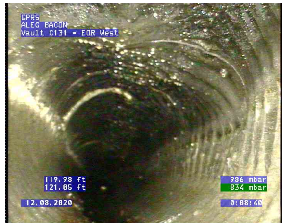
Vault C131 - EOR West_0011.bmp, , 120.01ft Deformed Horizontal, 10% changed
