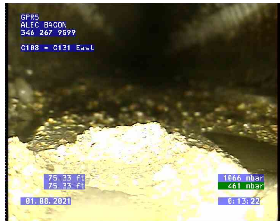
C108 - C131 East_0007.bmp, , 75.36ft Survey Abandoned / stuck in mud
