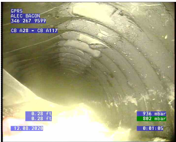
CB A28 - CB A117_0003.bmp, , 0.30ft Deformed, 15% changed, Start
