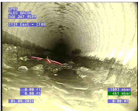
C131 East - C108_0000.bmp, , 0.00ft Water Level
