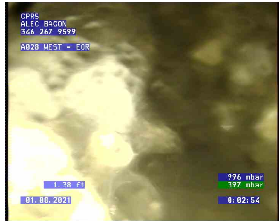
A028 WEST - EOR_0001.bmp, , 1.38ft Survey Abandoned / stuck in mud
