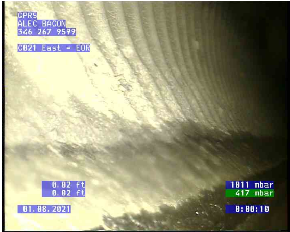
C021 East - EOR_0000.bmp, , 0.03ft Water Level
