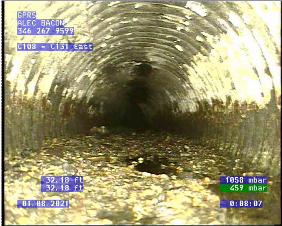
C108 - C131 East_0004.bmp, , 32.19ft Deposits Settled Gravel, 5% of cross sectional area from 4 o'clock to 8 o'clock, Start
