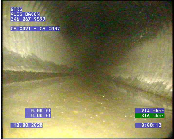
CB C021 - CB C002_0000.bmp, , 0.00ft Catch Basin
