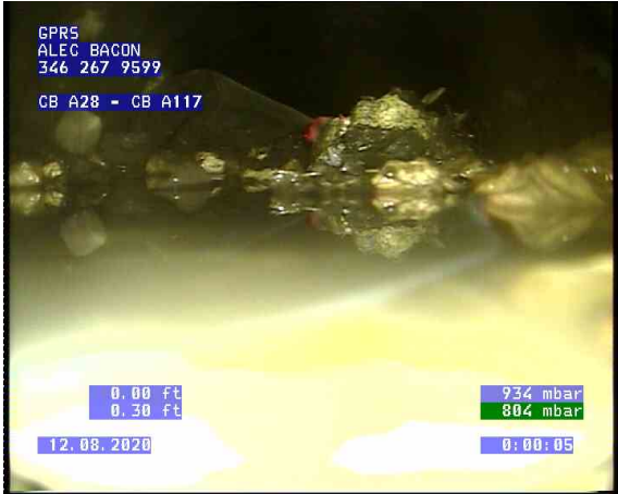
CB A28 - CB A117_0000.bmp, , 0.00ft Catch Basin
