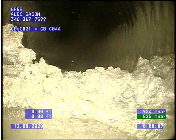
CB C021 - CB C044_0000.bmp, , 0.00ft Catch Basin
