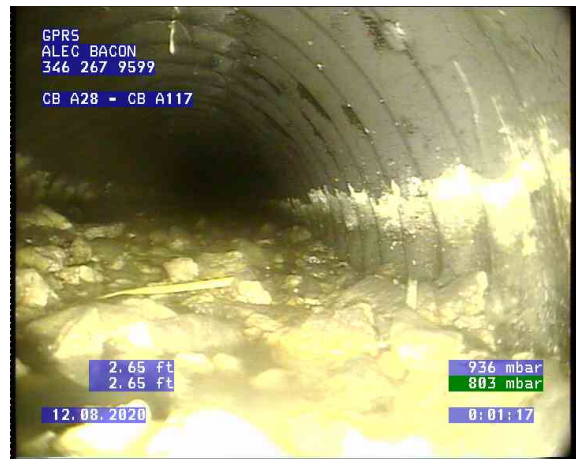
CB A28 - CB A117_0004.bmp, , 2.66ft Deposits Settled Compacted, 15% of cross sectional area from 5 o'clock, to 7 o'clock, Start
