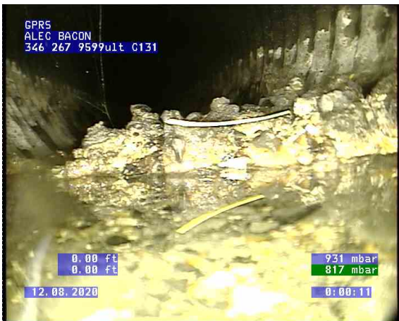
CB C065 - Vault C131_0001.bmp, , 0.00ft Water Level
