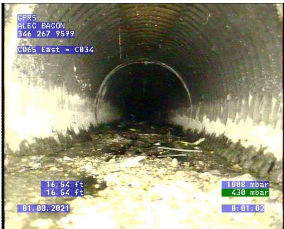
C065 East - C034_0002.bmp, , 16.54ft Deposits Settled Gravel, 5% of cross sectional area from 5 o'clock to 7 o'clock, Start
