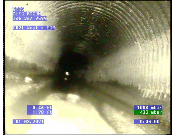
C021 West - EOR_0002.bmp, , 0.46ft Survey Abandoned / stuck in mud
