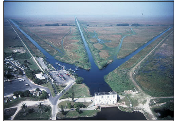
Figure 11. An extensive system of canals, levees, and water control structures has modified Everglades water conditions and provides an inadvertent conduit for pollutant transport. The S9 pump station (foreground) in Broward County discharges stormwater westward from an urban basin into the Everglades (background).
