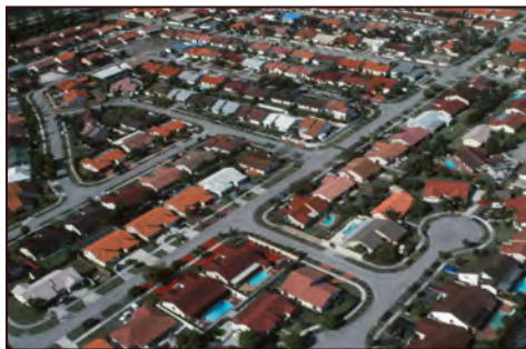
Figure 7. Residential development on former Everglades wetlands in western Dade County, 2005.
