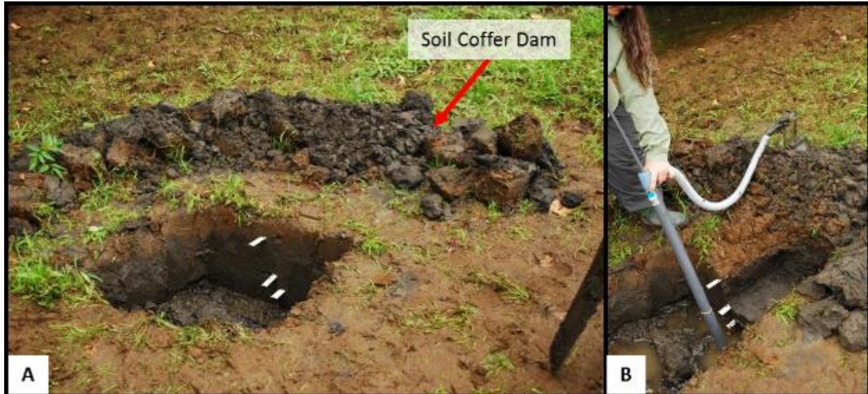
Figure 6-10. Techniques for sampling submerged or saturated soils. A) Soil coffer dam surrounding the Soil Pit. B) Use of a hand pump to remove water from the Soil Pit. Photos by Gregg Lomnicky.
