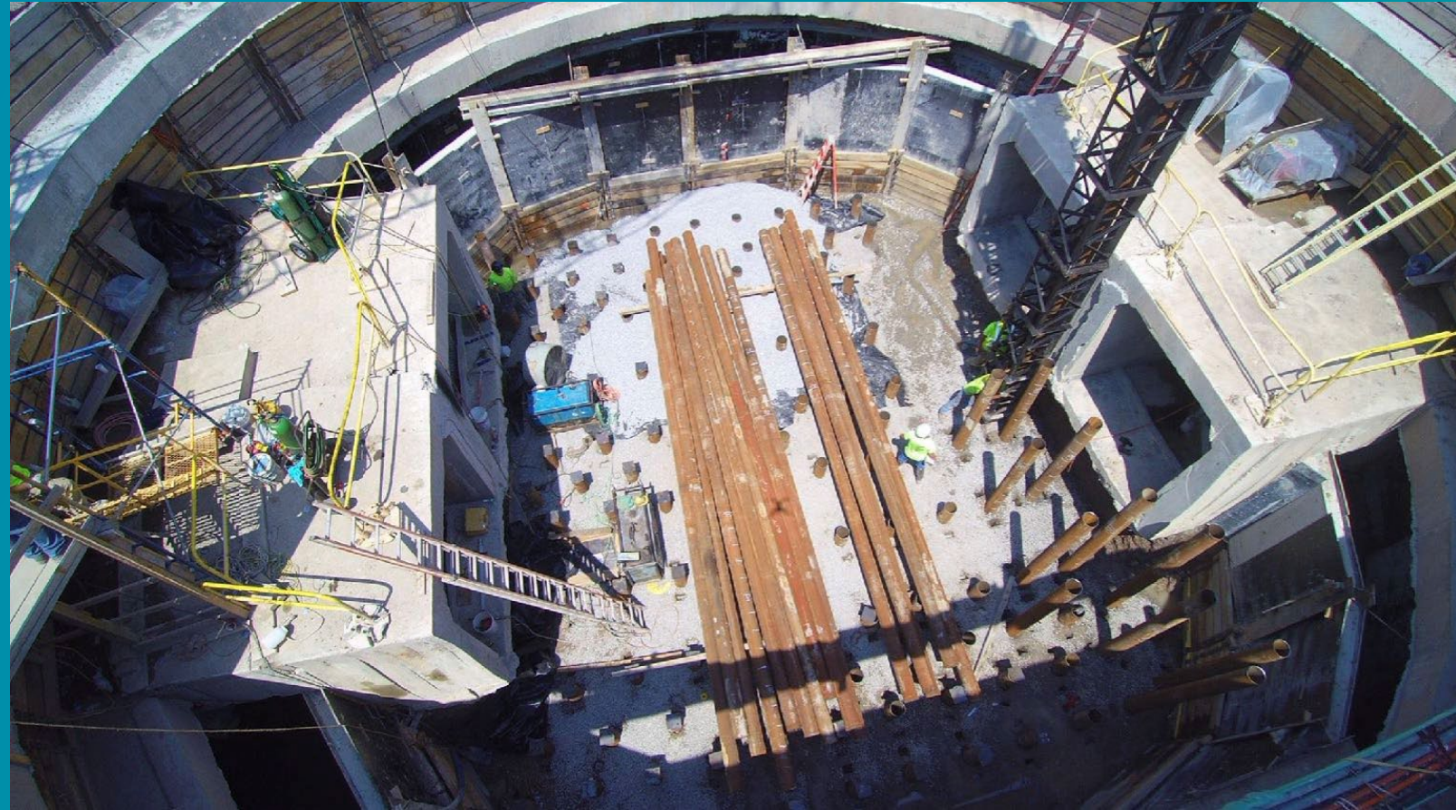
Herchel at Deer RTC Construction Fall 2019 Commissioned January 2020
