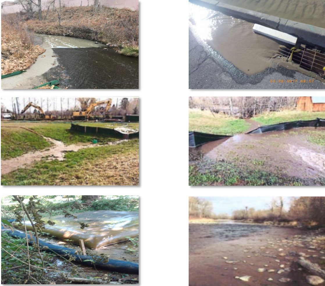
Figure 1. Photos depicting dewatering discharges from permitted construction sites.
