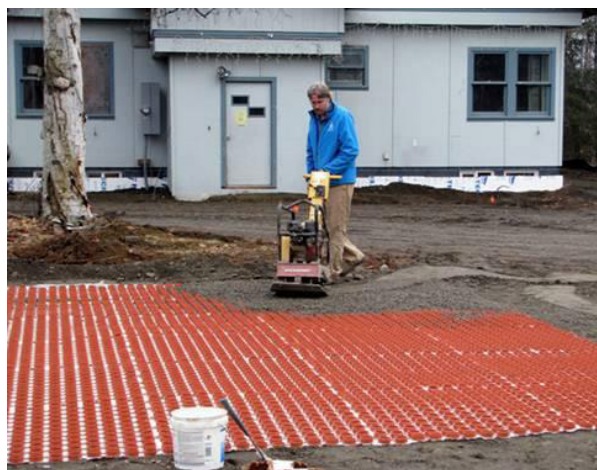
Figure 2. A Kenai Watershed Forum staff member applies the last layer of gravel on a new GravelPave2 system in front of the historic Soberg House at the confluence of Soldotna Creek and the Kenai River.
