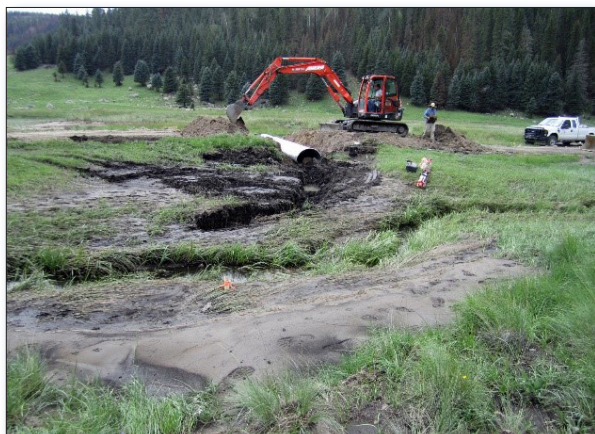
Figure 2. Improving a road crossing reduced erosion at the confluence of Rio de los Indios and San Antonio Creek.
