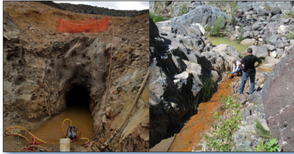
Figure 4. Before remediation, the adit discharged about 2.6 million gallons of contaminated water annually.
