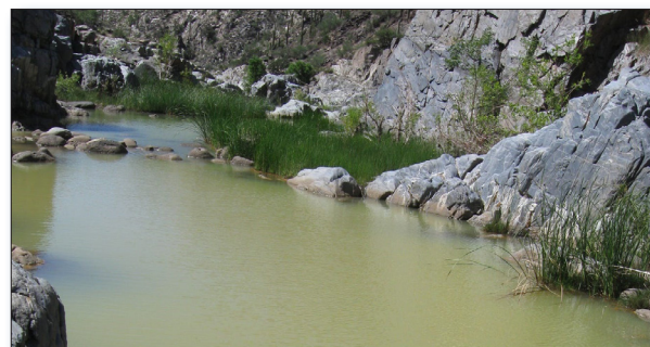
Figure 3. A discolored Boulder Creek flows near an eroding tailings pile (before remediation).
