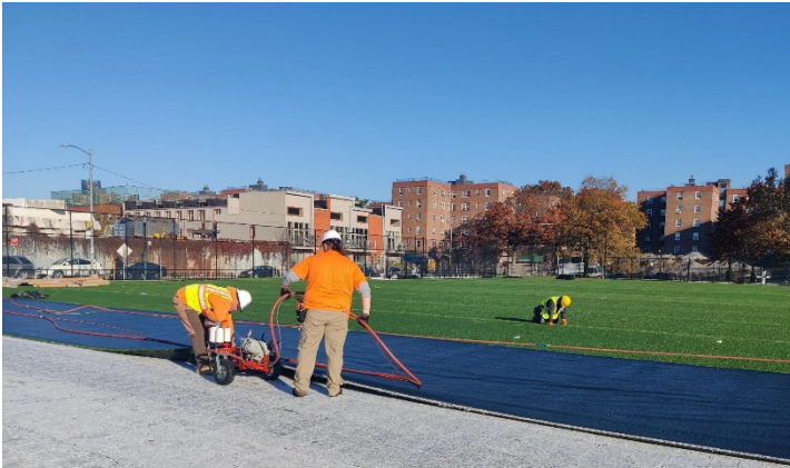
Contractors installing artificial turf on Ball Fields 5 - 8
