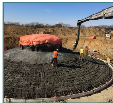
Pouring base of wind turbine
