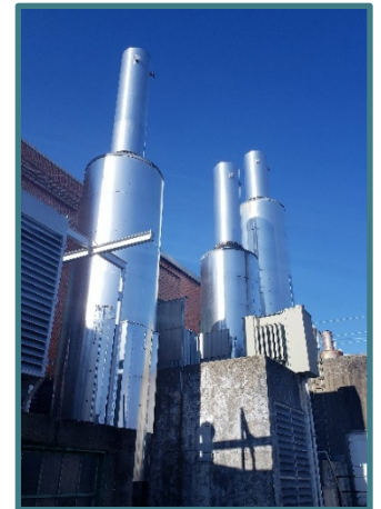
CWEP new exhaust stacks housing catalytic converters
