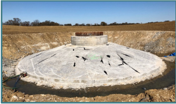
Completed base of wind turbine
