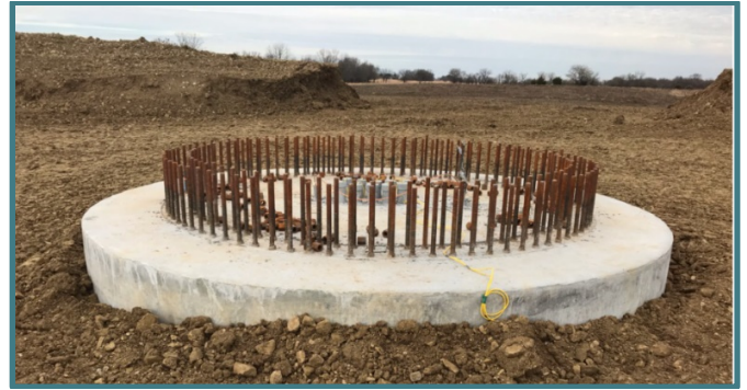
Graded base where wind turbine will attach
