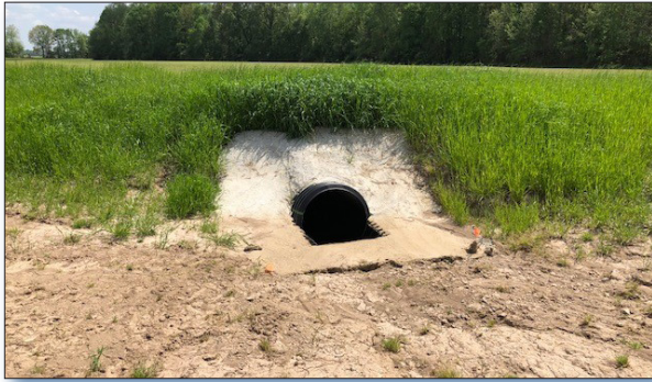
Figure 3. Close-up of a grade stabilization structure.
