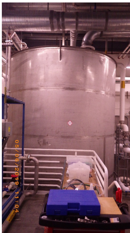
Figure 7 - Building 11, DRP Equalization Tank, 12,000-L
