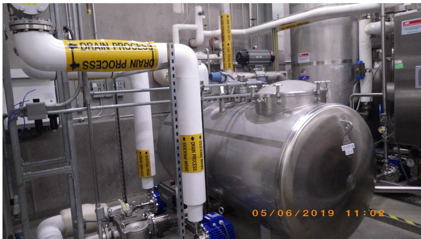
Figure 6 - Building 11, DRP Sump Tank-1,000-L
