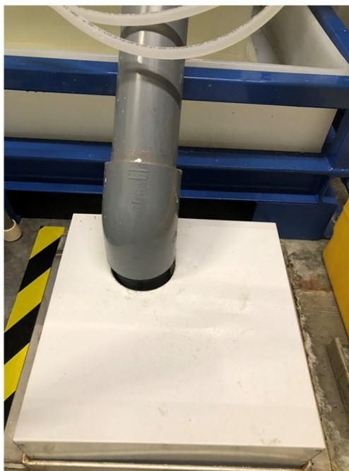
Figure 10 - Outfall 001-Discharge from pH Neutralization Skid in Building 11
