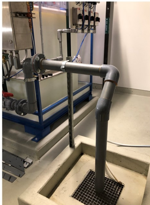
Figure 12 - Outfall 002, Discharge from pH Neutralization Skid in Building 16
