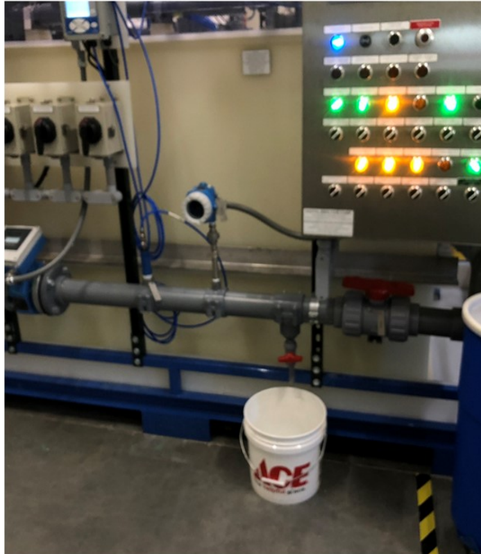
Figure 9 - Building 11, pH Neutralization Skid
