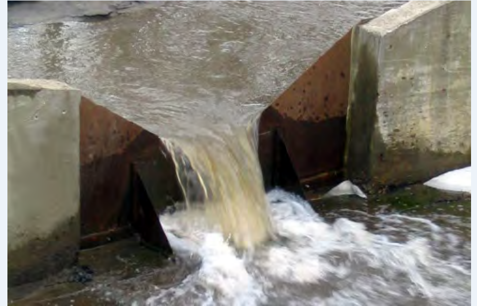
120° V-notch weir, Englesby Brook, Burlington, VT (USEPA 2016)
