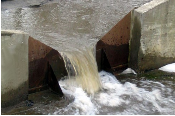
120° V-notch weir, Englesby Brook, Burlington, VT (USEPA 2016)
