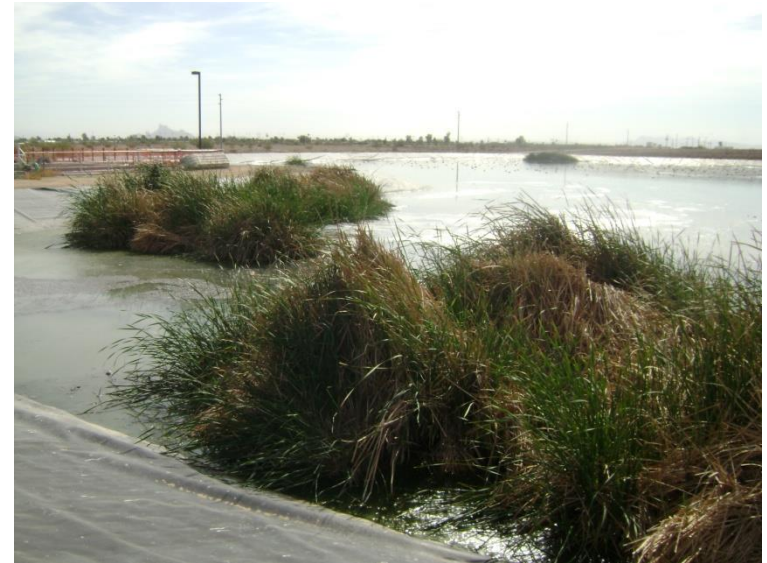
If not removed, cattails and rushes can cause solids accumulation as they die and decay. These cattails are growing on top of accumulated sludge.
