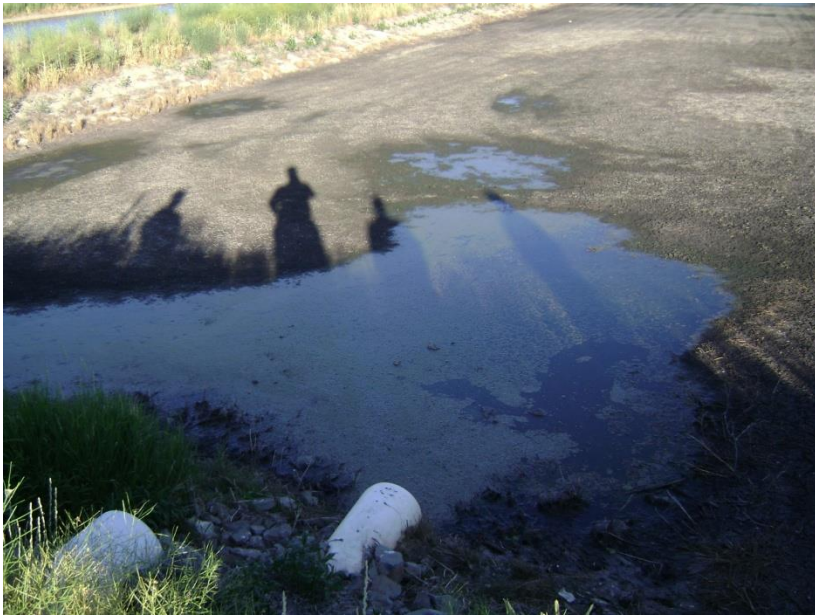
Solids Leaving the lagoon Can Cause Clogging of Perc Basins
