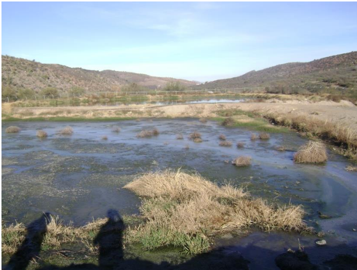
Solids Leaving the lagoon Can Cause Clogging of Perc Basins
